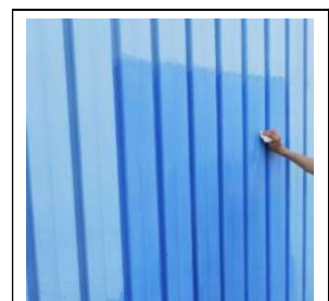
20 years old industrial facade painted metal profiles. Treated with: MPS REFRESH. After rubbing in twice.
